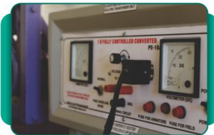
Control of Electronic Drive Lab
